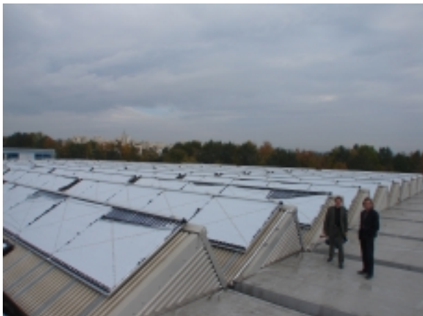
Car industry, 1330 m 2 CPC-collector for solar cooling and heating near Stuttgart, Germany
